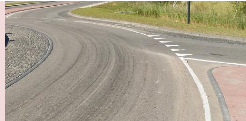
Example of 1.13 marking in roundabouts (Lithuania)
