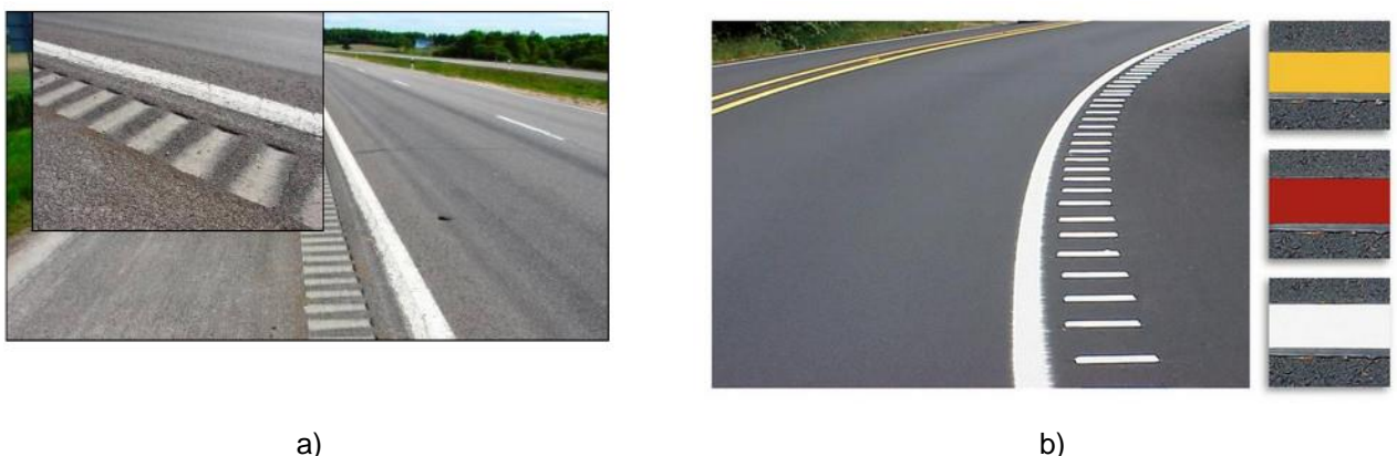
Figure 5-8. a) milled rumble strip; b) thermoplastic rumble strip
